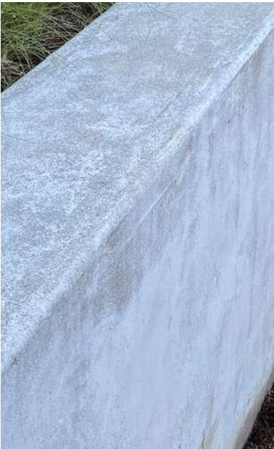
Concrete edging/ retaining
